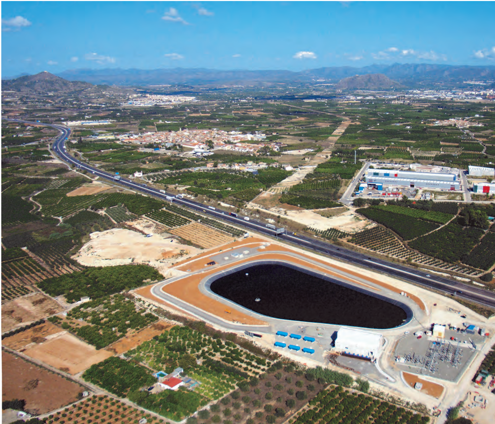
Image: Pool and pumping station of the Júcar-Vinalopó pipeline at Llanera de Ranos
